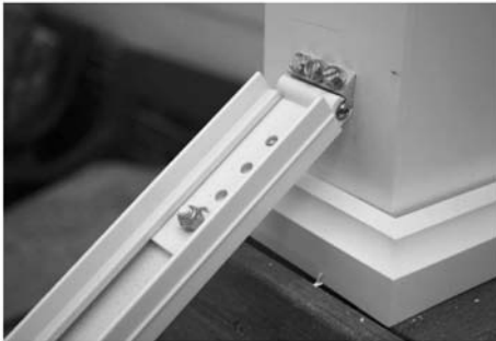
Photos 13C & 13D: INSERT SIDEWALK BOLTS & INSTALL LOCK NUTS
