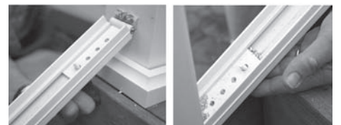
Photos 13A – 13D: INSERT SIDEWALK BOLTS & INSTALL LOCK NUTS
