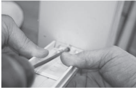
Photo 10B: DRILL PILOT HOLES FOR \frac{1}{4} " HEX HEAD SCREWS – BOTTOM OF STAIRS
