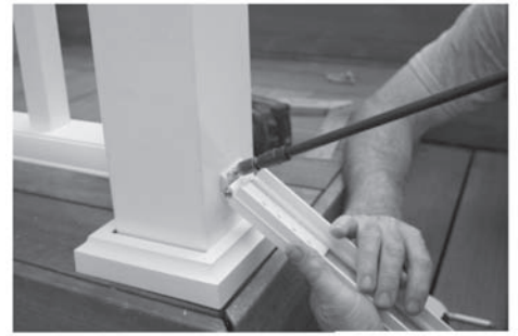
Photos 11A & 11B: DRIVE HEX HEAD SCREWS INTO NEWEL POST
