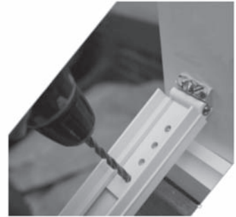
Photos 12A & 12B: DRILL MOUNTING BRACKET BOLT HOLE THROUGH ALUMINUM STIFFENER
