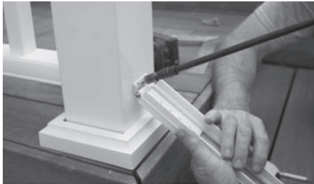
Photos 11A & 11B: DRIVE HEX HEAD SCREWS INTO NEWEL POST
