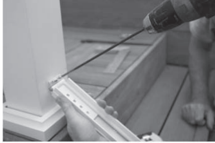
Photo 10B: DRILL PILOT HOLES FOR \frac{1}{4} " HEX HEAD SCREWS – BOTTOM OF STAIRS
