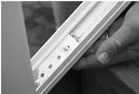
Photos 13C & 13D: INSERT SIDEWALK BOLTS & INSTALL LOCK NUTS
