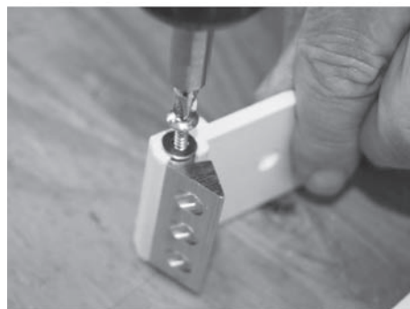
Photo 7C: SECURE LEAF IN PLACE WITH SCREWS
