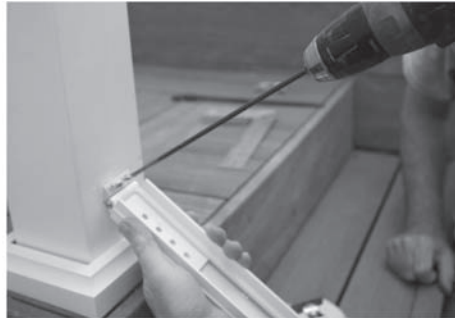
Photo 10B: DRILL PILOT HOLES FOR \frac{1}{4} " HEX HEAD SCREWS – BOTTOM OF STAIRS
